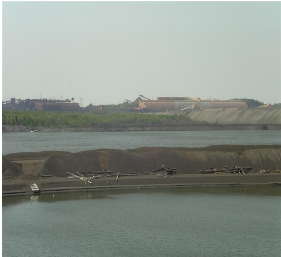
Tailings ponds and taconite processing facilities at Minntac, MN
