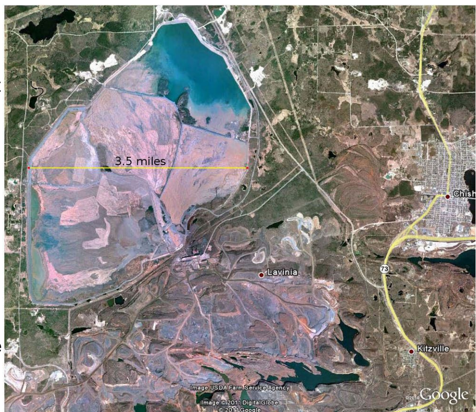
Hull-Rust-Mahoning (Hibbing) tailings basin, MN
